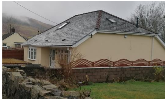
Fig 6 (below): Side elevation of adjacent property.
