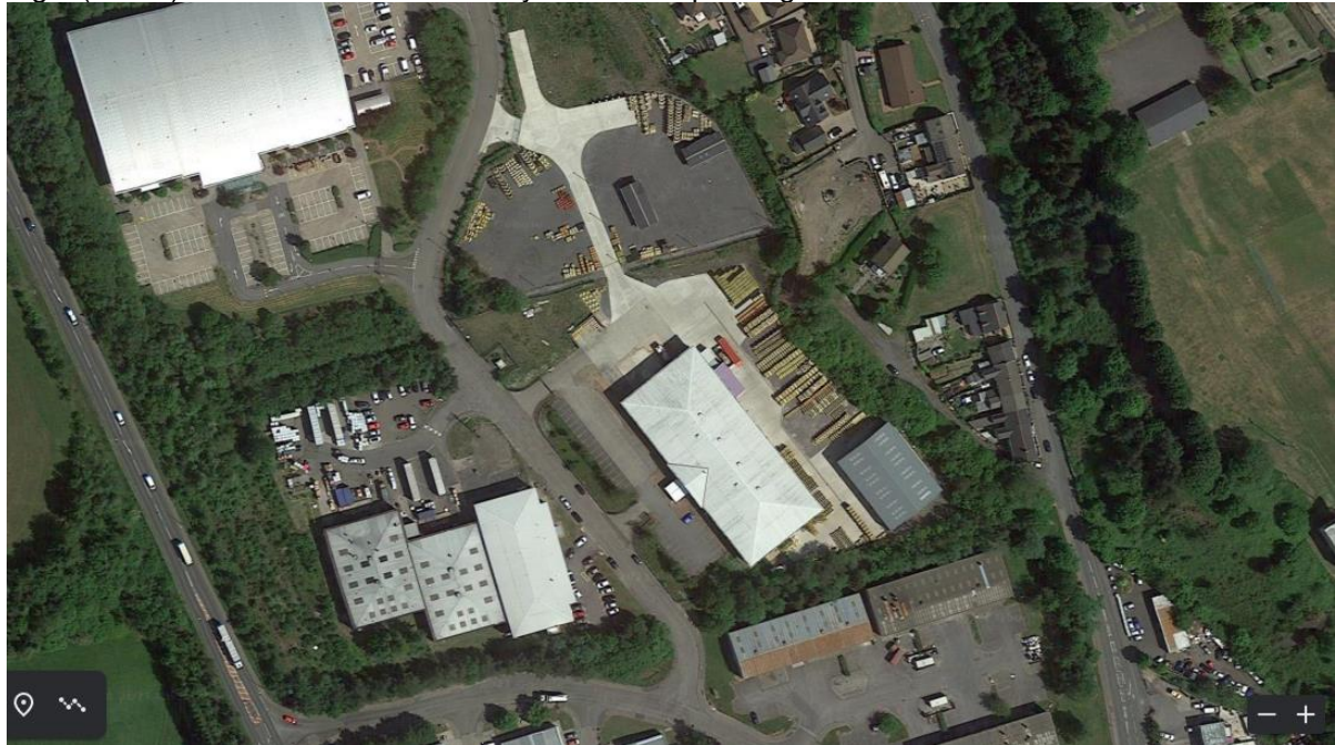
Fig 6 (Below): Industrial estate bound by dense tree planting
